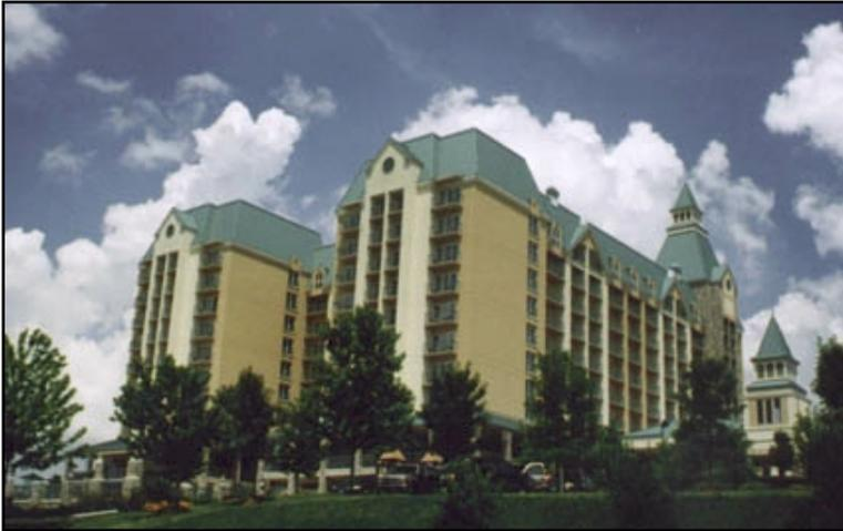
Erection played a big part in the decision between concrete and steel. The 48 inch (1.22 m) deep lightweight concrete double tees were priced against fire-proofed structural steel. Because the precast long-span convention roof double tees could be erected at the same time the two bays of floor tees and supporting beams, columns, and wall panels were being erected, there were significant logistic advantages to the all-precast system.
